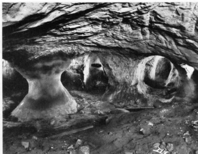
London Road mine: this view illustrates the high extraction ratio obtaining at this site, well below 25% of the rock being left in-situ to support the roof. A great deal of introduced or run-in soil and building rubble can be noted. Eighteenth-century and earlier pottery has been reported, although nothing has been satisfactorily archaeologically recorded because during a lengthy period when there was unrestricted access collectors of Victorian and earlier bottles dug extensively for additions to their collections. Clay tobacco pipes dated to the period 1730 – 1780 have also been reported.
